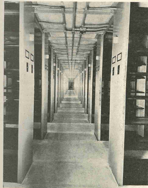
Looking down an aisle on one of the floors in the stack room. The arrangement of the shelves, the electrical fixtures and the rows show well in this illustration. The stack room, when finished, will house more than 1,500,000 books.
