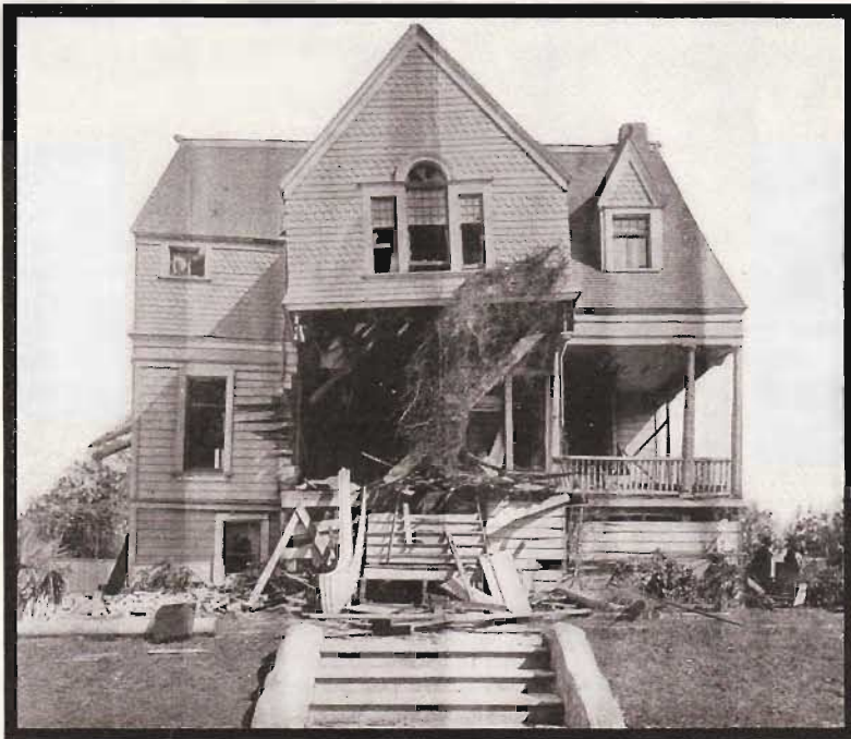
FRONT VIEW OF THE GALLAGHER HOUSE, SHOWING WRECK CAUSED BY DYNAMITE
