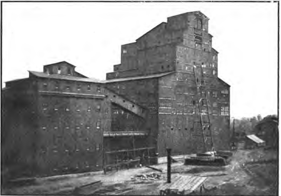
ONE OF THE BETTER COAL BREAKERS.
