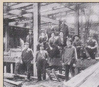
Members of Local No. 33, Rochester, New York, on job for the Genesee Bridge Company.
