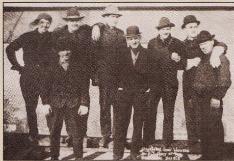
Members of Local No. 86, Seattle, Washington, on the 36th story of the Smith Building.
