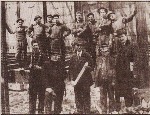
Gang on job of Snead Architectural Iron Works at Nashville, Tennessee, in 1913.
