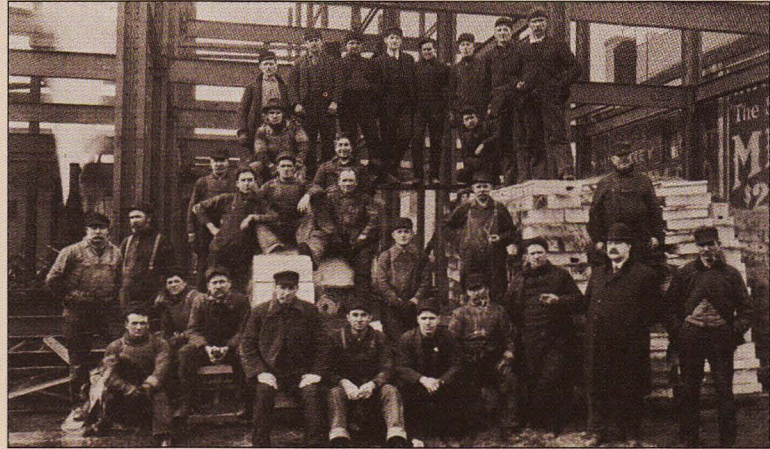
A bunch from Local No. 8, who are erecting building for Charles Volkmann & Company
