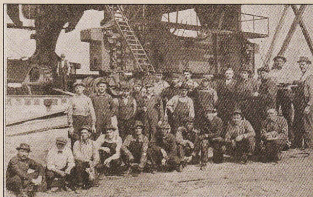
Members of Local No. 45, Jersey City, New Jersey employed on Ore Dumper for the Lehigh Valley Railroad at Bayonne, New Jersey.
