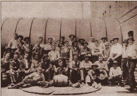
Enameled tanks being installed with members of Local No. 11, Newark, New Jersey.
