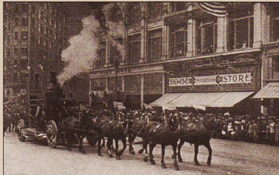
Complete pile-driving outfit used as a float in the Labor Day parade by Local No. 77 of San Francisco, California.
