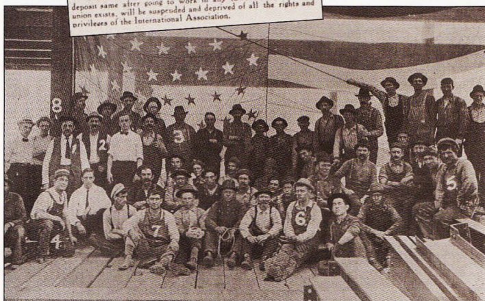
Members of Local No. 1, Chicago, working on the Peoples Gas Light and Coke Co. building.
