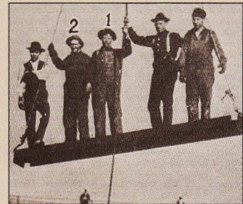
Members of Local No. 24, Denver, erecting Auditorium where the Democratic Convention was held in 1908.
