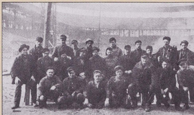
Members of Local No. 44, Cincinnati, Ohio, working on the new ball park.
