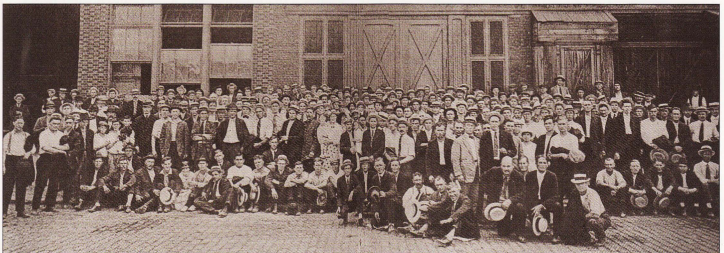
Two hundred and fifty Ironworkers from Locals No. 189 and 189A of New York, New York and Jersey City, New Jersey somewhere in France to build docks and piers for the U.S. Government.
