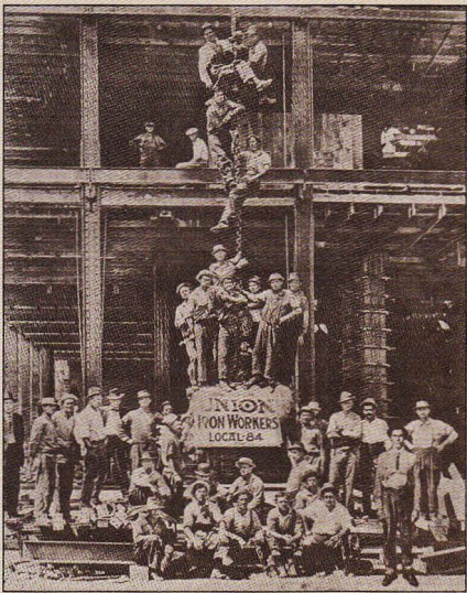
Members of Local No. 84, Houston, Texas, who erected the 13 story Texas Oil Company Building in Houston, Texas.
