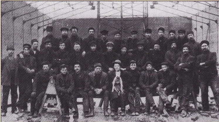
Members of Local No. 4, Toronto, Canada who are erecting work at the gas plant for the Dominion Bridge Company.
