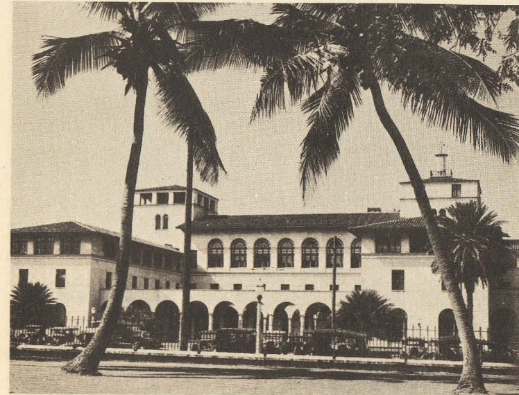
The Federal Building in Honolulu
