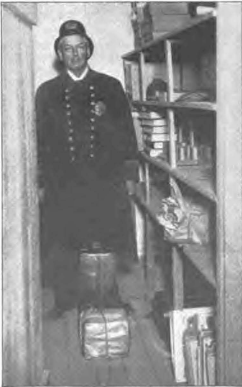
DYNAMITE FOUND IN THE VAULT OF THE IRON-WORKERS' UNION AT THEIR HEADQUARTERS IN THE AMERICAN CENTRAL LIFE BUILDING, INDIANAPOLIS
