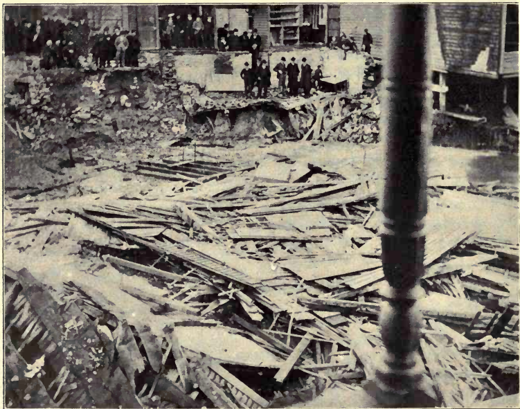
SCENE OF A CAVE-IN ON LACKAWANNA STREET, OLYPHANT, JANUARY, 1902. (Four houses, a barber shop and a hotel were swallowed up within an hour of the first warning.)
