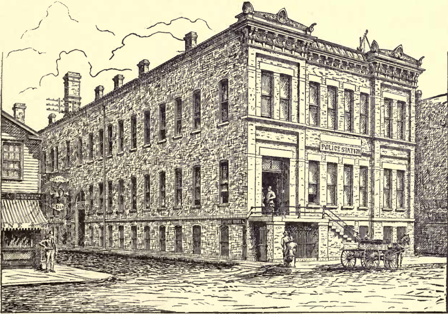
THE DESPLAINES STREET STATION.
